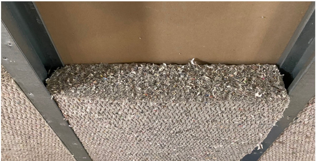
Figur B4.2 iCell-skiva mellan Gyproc XR70.
